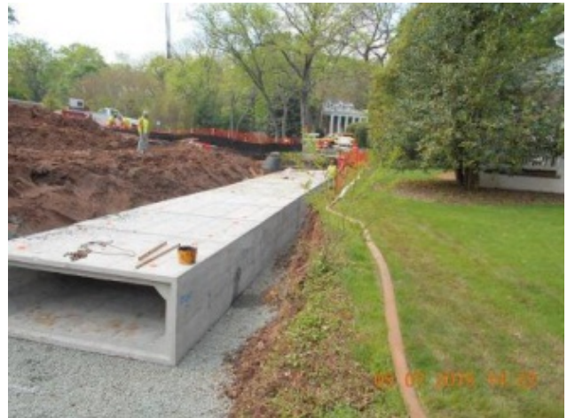
Upper Flat Branch Interceptor Project
